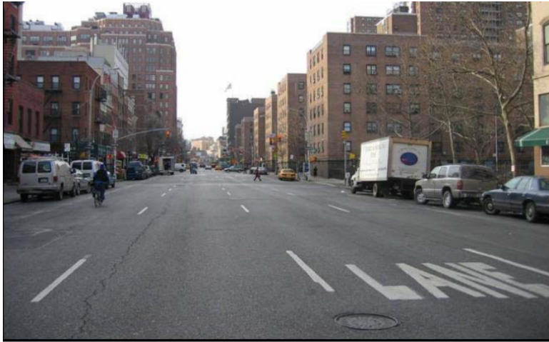
Figure 2: Ninth Avenue Before and After Changes
