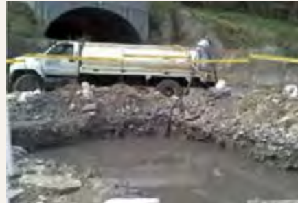
Figure 21 and 22: Water catchment areas were excavated to store runoff or surface waters for later use during construction / Source: CONNET, "El proyecto mantendrá la calidad del agua," photo report, n.d.
