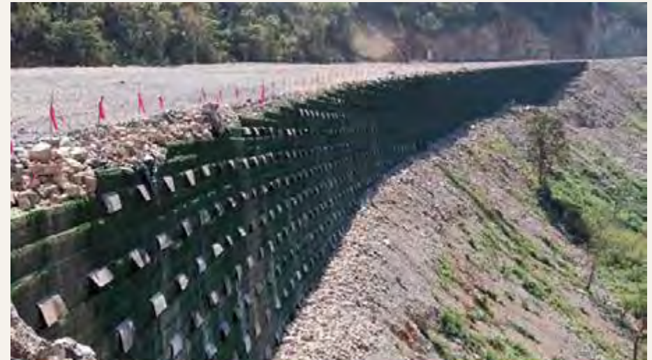
Figure 15: Wall reinforced with geosynthetics / Source: ICA, Globalvía, FCC Construcción, AUNETI, and CONNET, Mexico City-Tuxpan Highway: Nuevo Necaxa-Tehuacán (Mexico: ICA and Global Via Infrastructures, 2011), 121.
