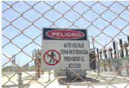
Figure 04: Sign reading “Danger: High Voltage Restricted Zone Access Prohibited” / Source: EGE Haina.
