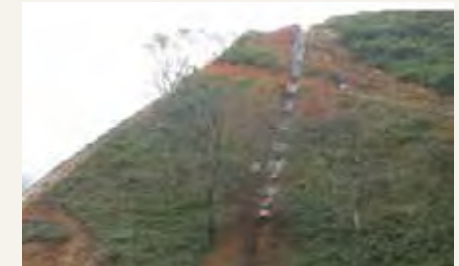
Figure 27–28: Drainage systems were implemented to control runoff and maintain the hydrological system / Source: CONNET, “El Proyecto Mantendrá la Conexión Hidrológica de la Zona,” photo report, n.d.
