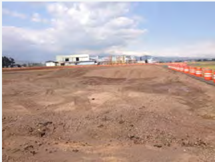
Figure 18: Re-use of excavated material /Source: Picture taken during onsite visit, April 2013 Figura 18: Reúso del material excavado / Fuente: Fotografía tomada durante la visita al sitio, Abril 2012
