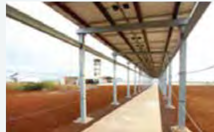
Figure 15 - 16: Use of solar panels to shade some of the external paths / Source: Energy and Atmosphere, L-13-3; credit SS- 7.1 , EA-2. Figura 15 - 16: Uso de paneles solares para dar sombra a pasarelas exteriores / Fuente: Energía y Atmósfera, L-13-3; crédito SS- 7.1, EA-2.
