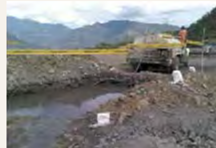
Figure 21 and 22: Water catchment areas were excavated to store runoff or surface waters for later use during construction / Source: CONNET, "El proyecto mantendrá la calidad del agua," photo report, n.d.
