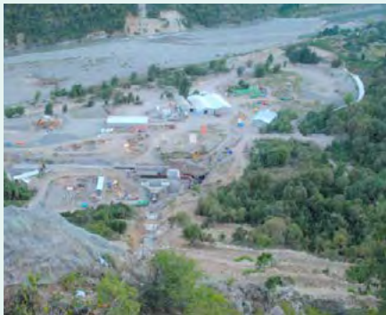
Figure 22: Deposits of accumulated material / Source: Besalco S.A. Figura 22: Depósitos de material acumulado / Fuente: Besalco S.A.
