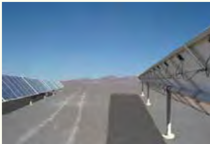
Figure 18: One of the Pozo Almonte solar photovoltaic plant / Source: SolarPack
