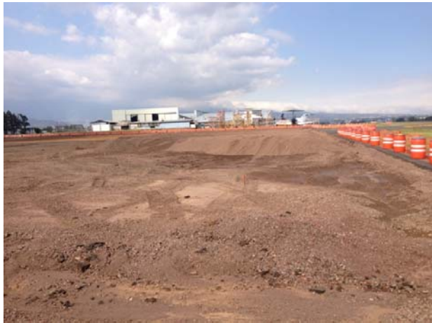
Figure 1: Re-use of excavated material
