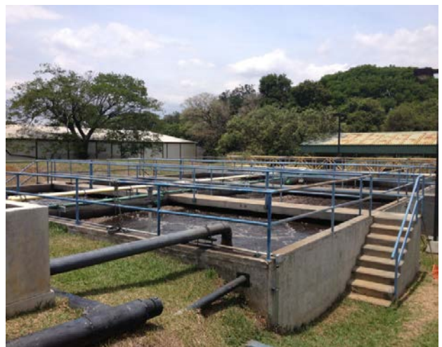
Figure 18: Water treatment plant.
