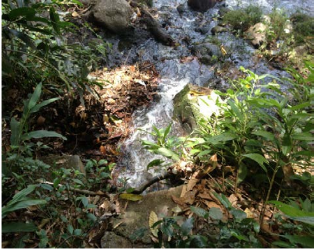
Figure 19: Discharge point of water treatment plant.
