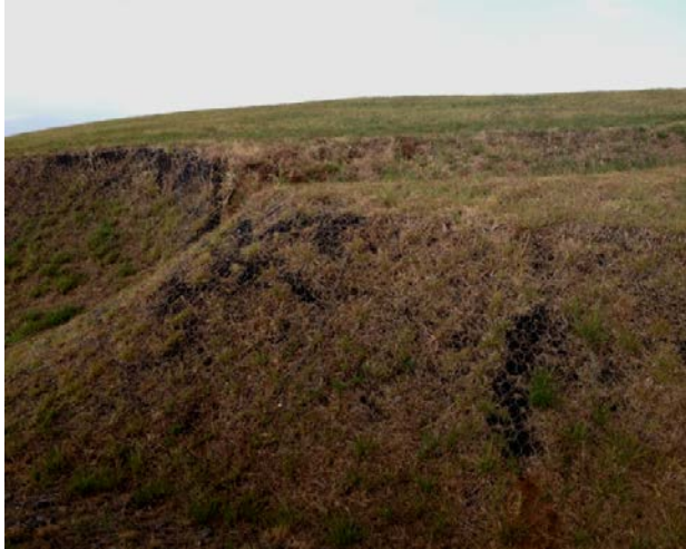
Figure 13: Prevention of embankments erosion.
