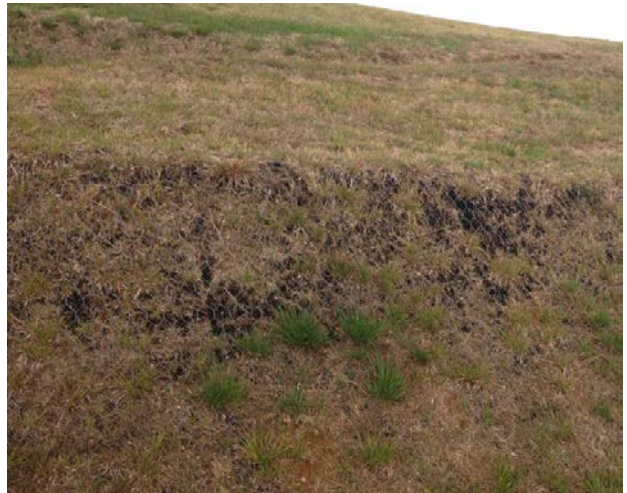
Figure 14: Prevention of embankments erosion
