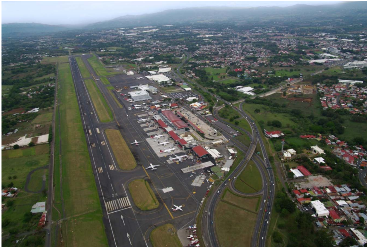
Juan Santamaría International Airport / Photograph provided by AERIS.
