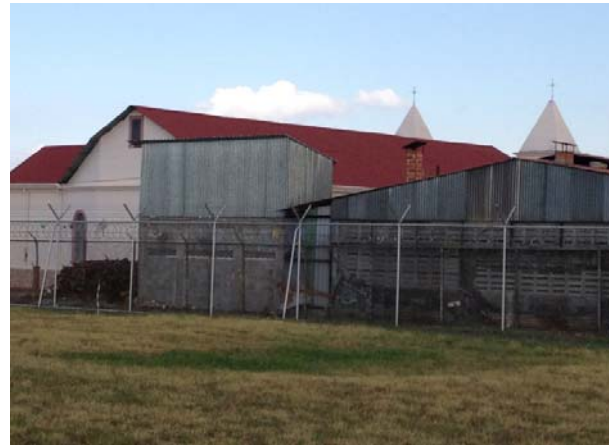
Figure 6: Church close to the airport.
