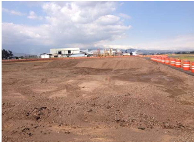
Figure 23: Re-use of excavated material. Source: Picture taken during onsite visit, April 2013
