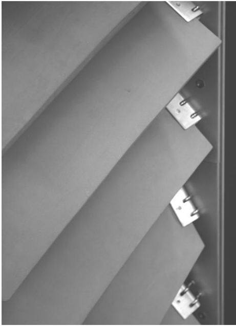
Fig. 8 High performance ceramic shading prototype
