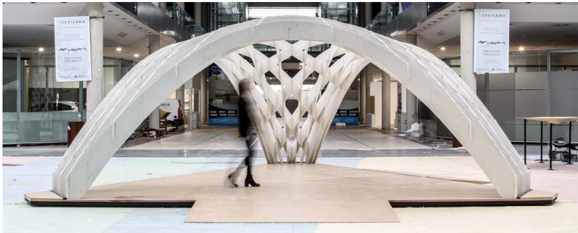
Figure 1: Ceramic tile grid shell installation
