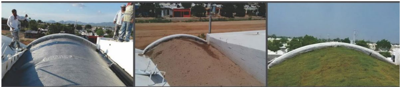
Green roofs used in the BOSCO development to mitigate radiation and energy consumption. Photo credit: Derex SA de CV.
