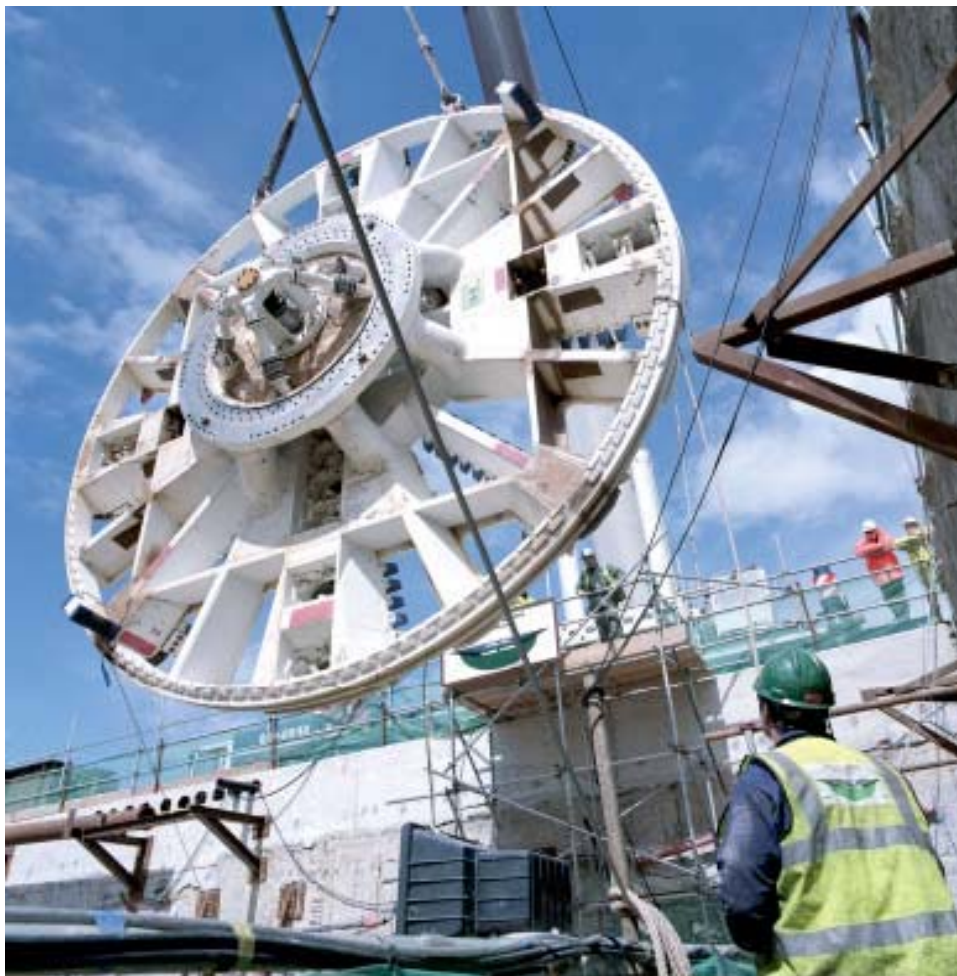
Figure 11: CTRL involved significant tunneling work
