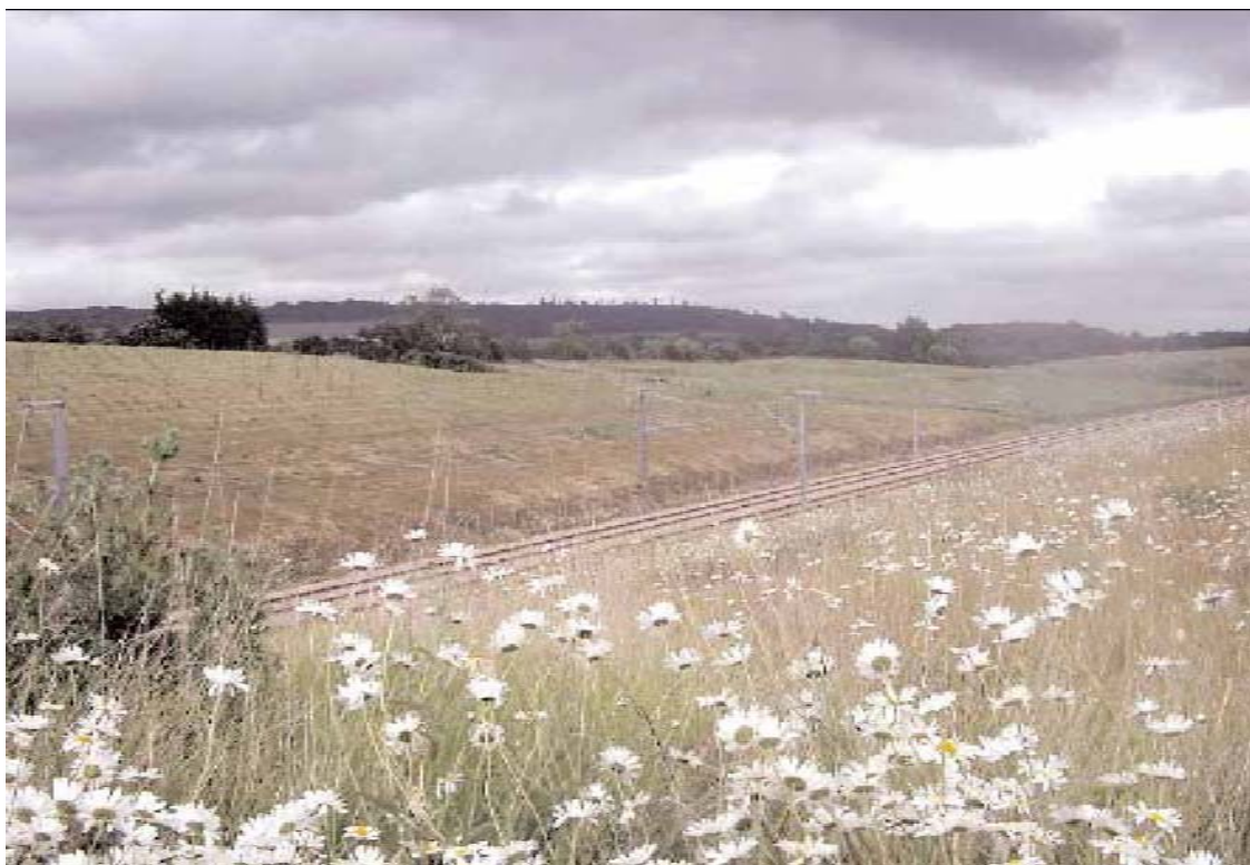
Figure 163: Section 1 of CTRL is finally complete
