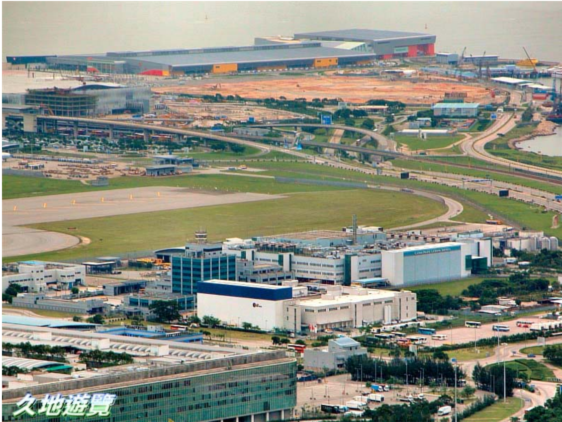
Figure 9. Sky City at Chep Lap Kok under construction. Courtesy Skyscrapercity.com.
