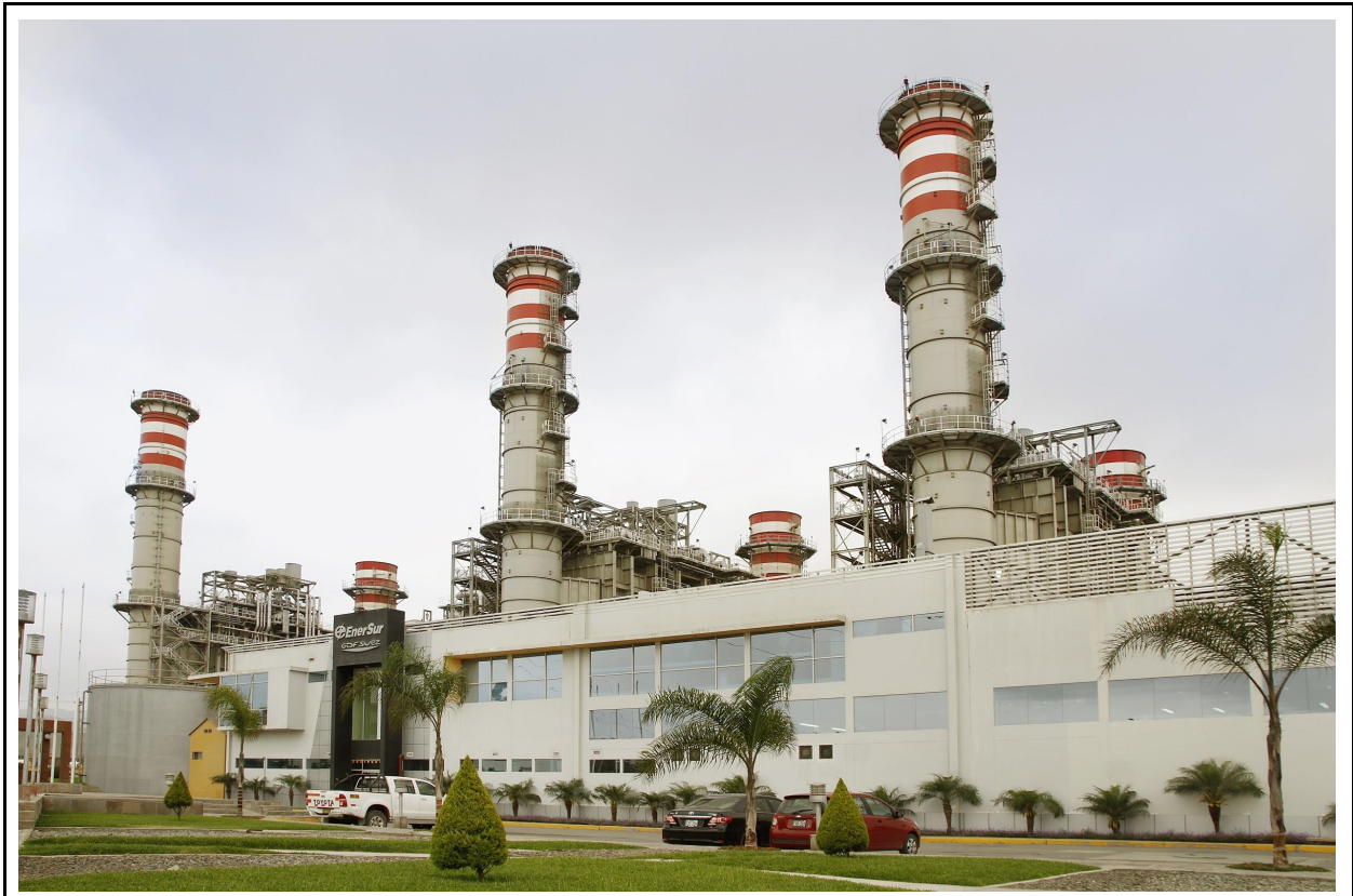
Figure 01: General view of the project.
