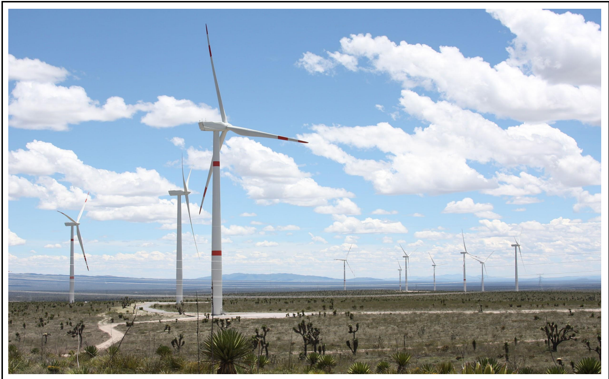
Figure 1: General view of the project Sources: Enel Green Power, "Evidencia Fotográfica [Photographic Evidence]"
