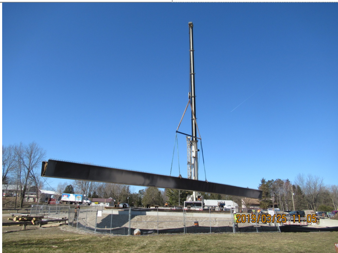
Fig.23: Supermodule and deck section
