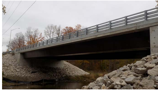
Fig.15: The new Bayfield River bridge
