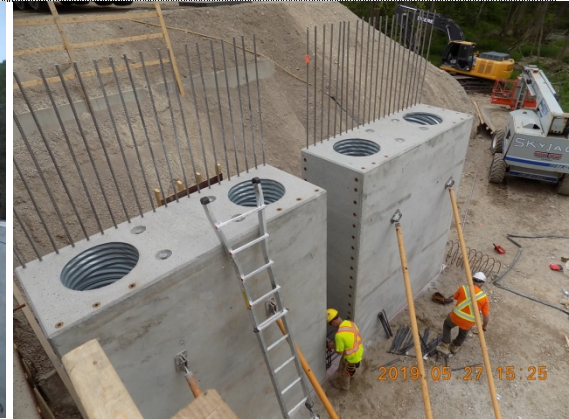
Fig.24: Precast abutments
