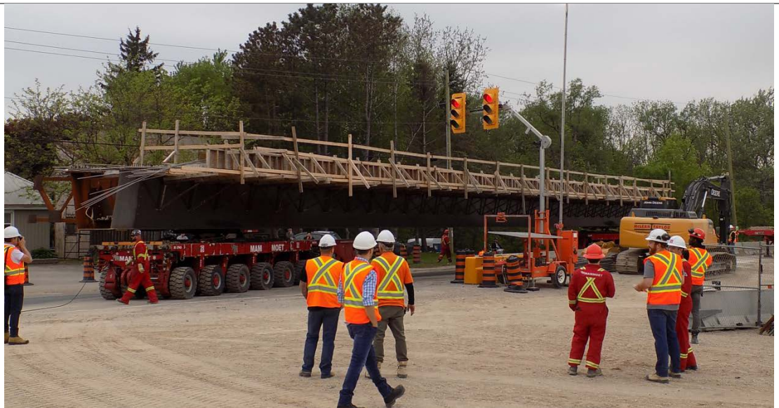
Fig.26: Transport of the supermodule from the temporary yard to the site with multi-axle hydraulic trailers with spacers
