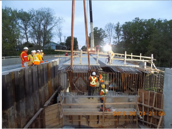
Fig.23: Supermodule and deck section
