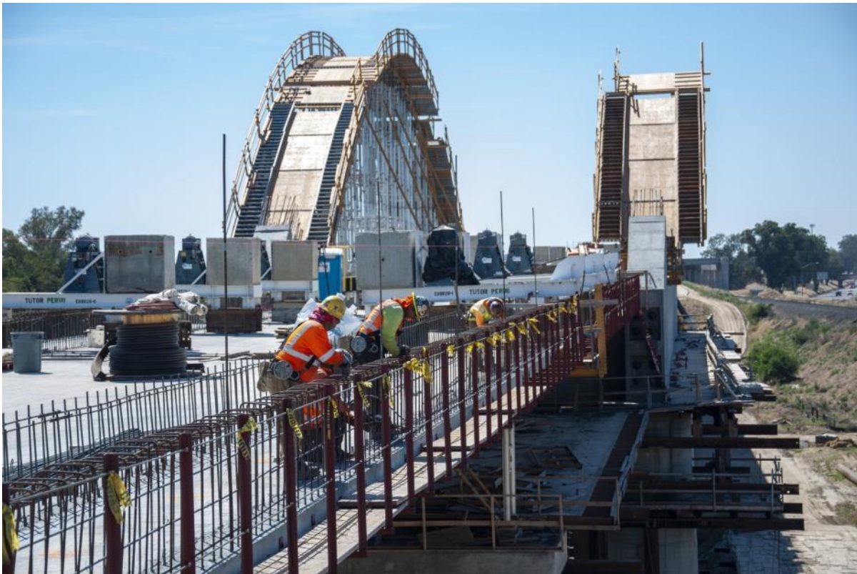
Fig. 62: San Joaquin river viaduct
