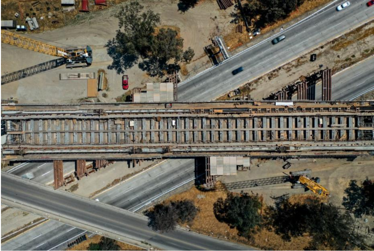
Fig. 63: Cedar Viaduct on April 2021 421
