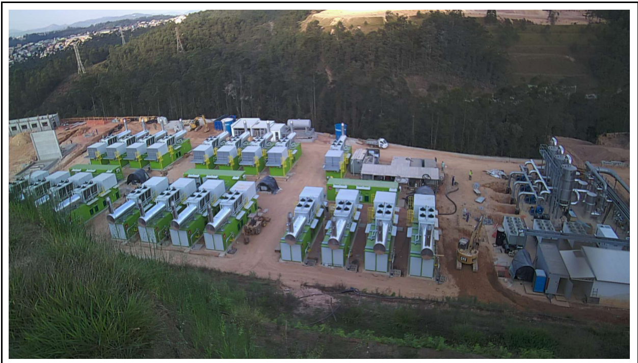
Figure 01: Aerial view of the biogas thermoelectric plant. Sources: Solví Valorização Energética.
