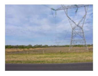
Figure 17: Easement strip of LEAT 500kV, clear and free from trees.
